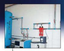
Distribution pipeworks in aluminium for compressed air, vacuum and other non dangerous gases, from 20 to 110 mm diameter.
